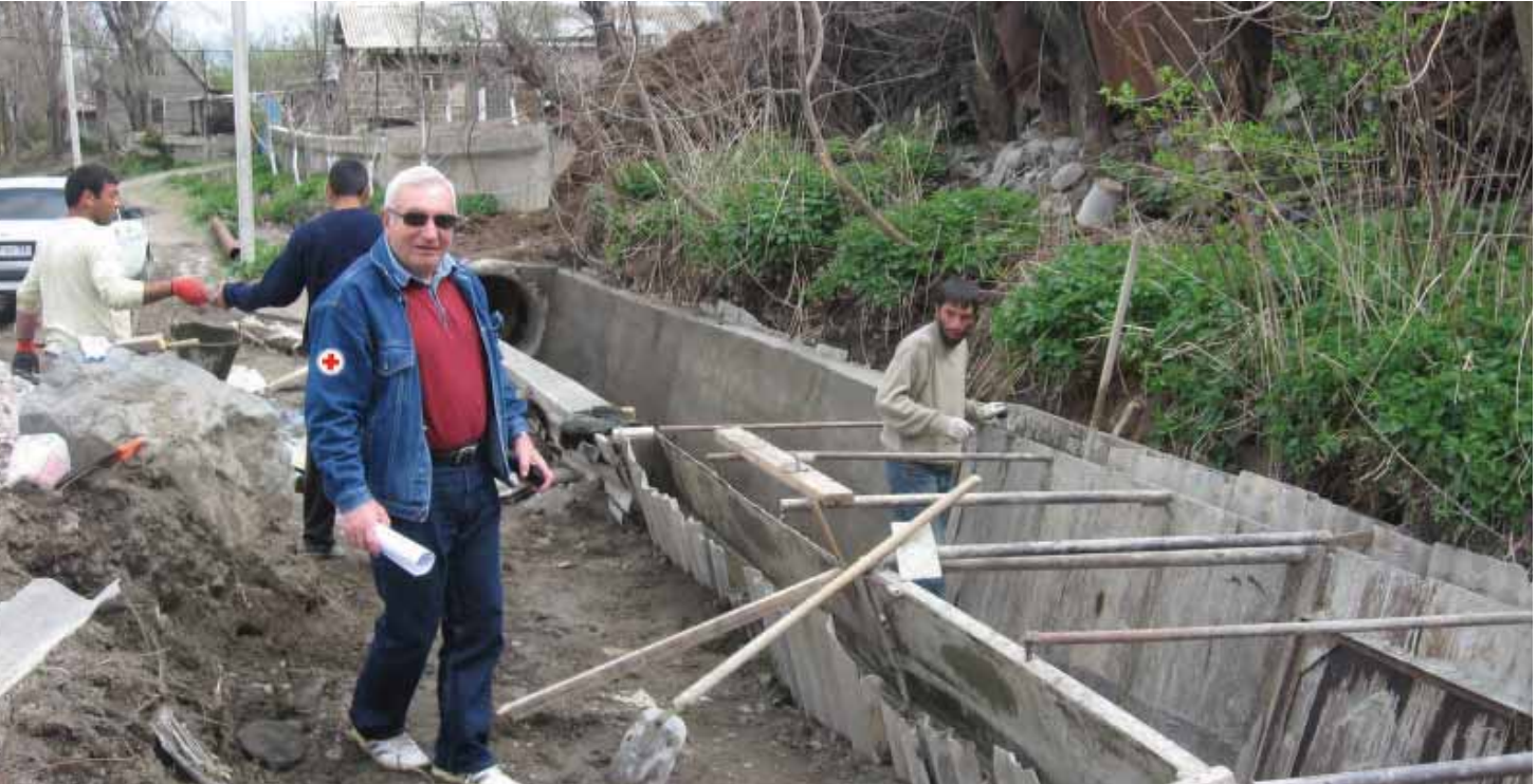
Support to mudflows cleaner construction, Lori, 2018
